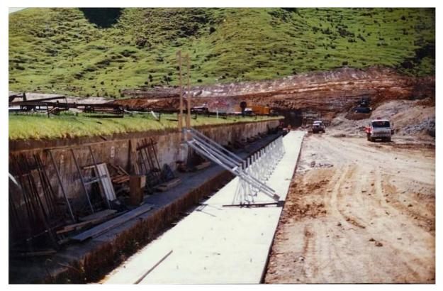
The new target hoists being erected on a new concrete platform. (NRANZ)
