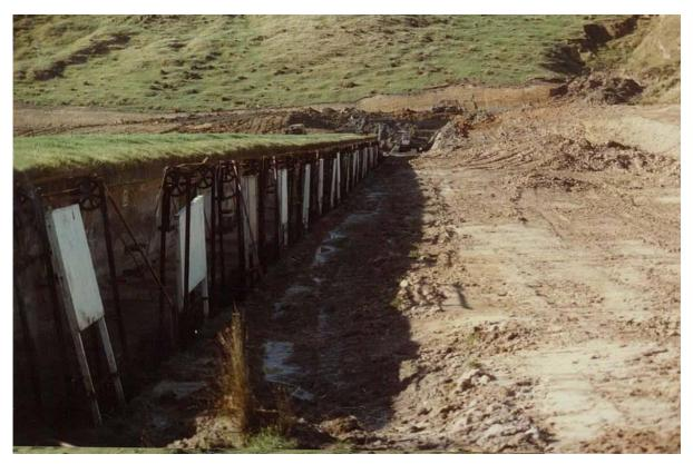
Seddon Range, 1984. The old Hythe pattern frames await removal as the area is prepared for new target hoists. Note the hillside partially removed to accommodate the extended range. (NRANZ)
